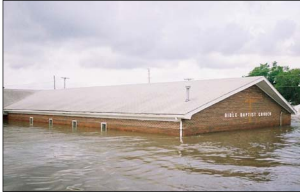
DISASTER: This photo of the main building was taken after the waters had abated over a foot (notice water line at top of windows).
